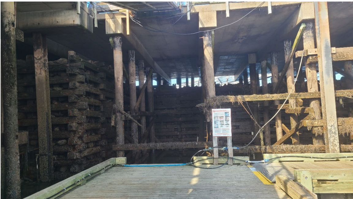
Figure 10: Southern End of Outer Approach Structure and Head of Wharf.
