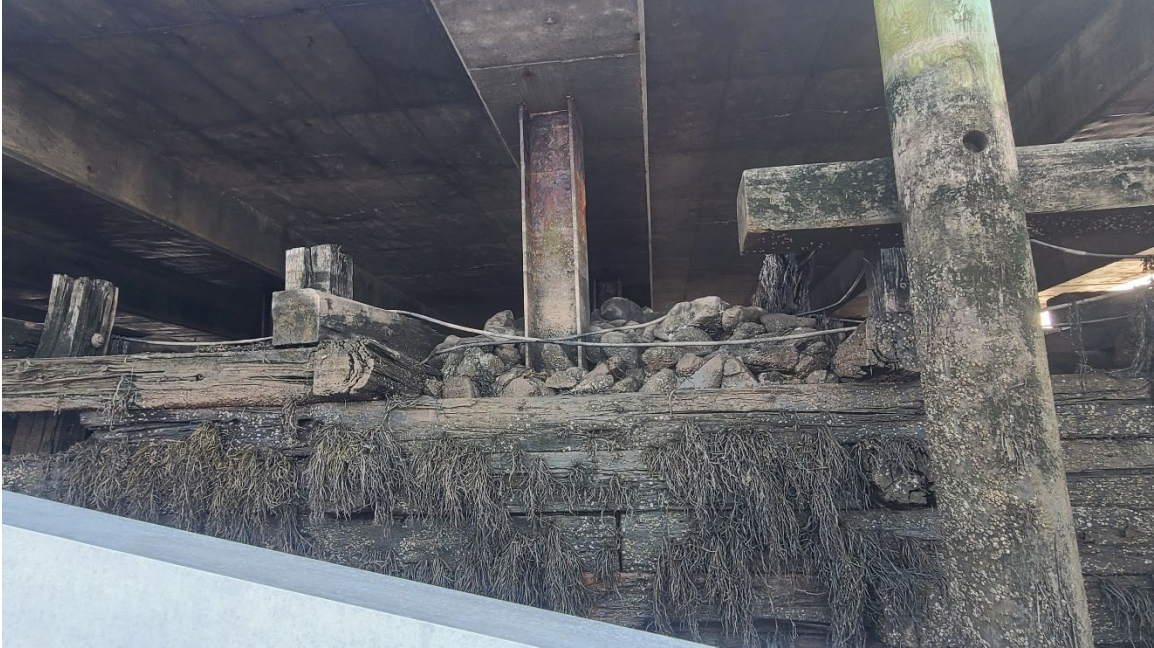
Figure 14: H pile at lines 11 – A and underside of deck in good condition.
