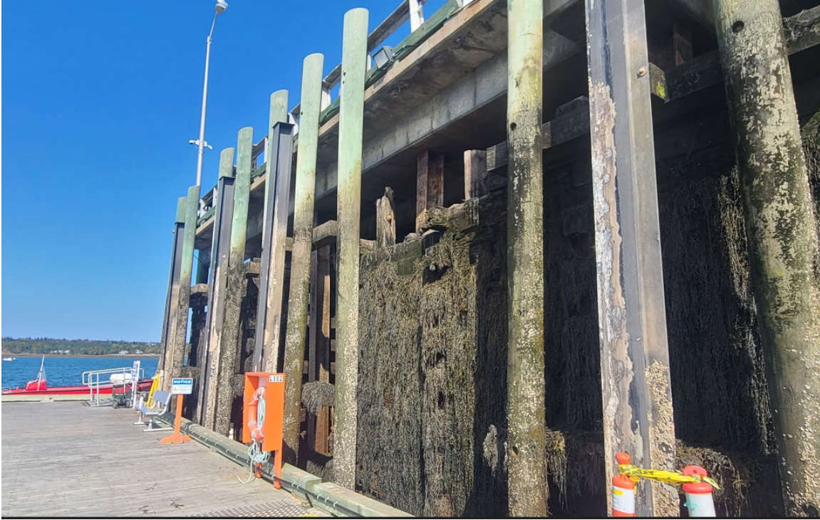
Figure 33: Timber Fender Piles and Steel H-Pile Guide Piles (South Face of Main Wharf)
