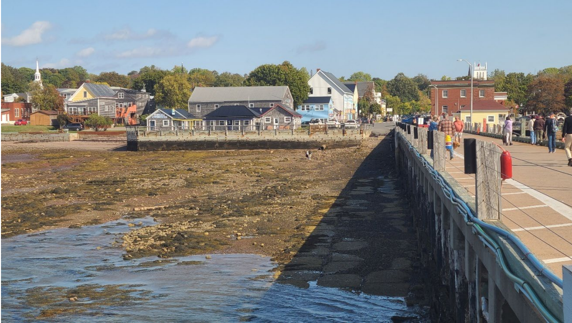
Figure 16: Utilities attached to Approach Structure.
