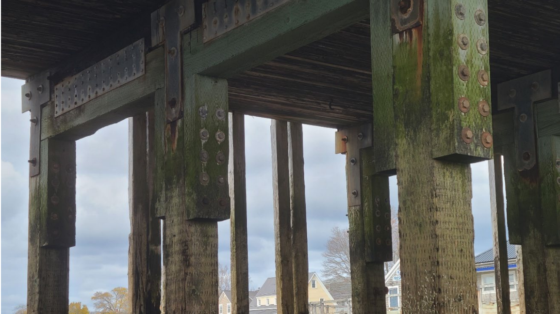
Figure 4: Typical repairs to pile bents.
