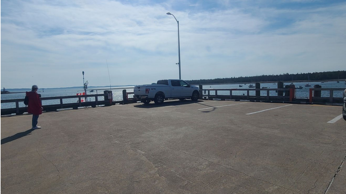
Figure 15: East end of wharf head deck in good condition.
