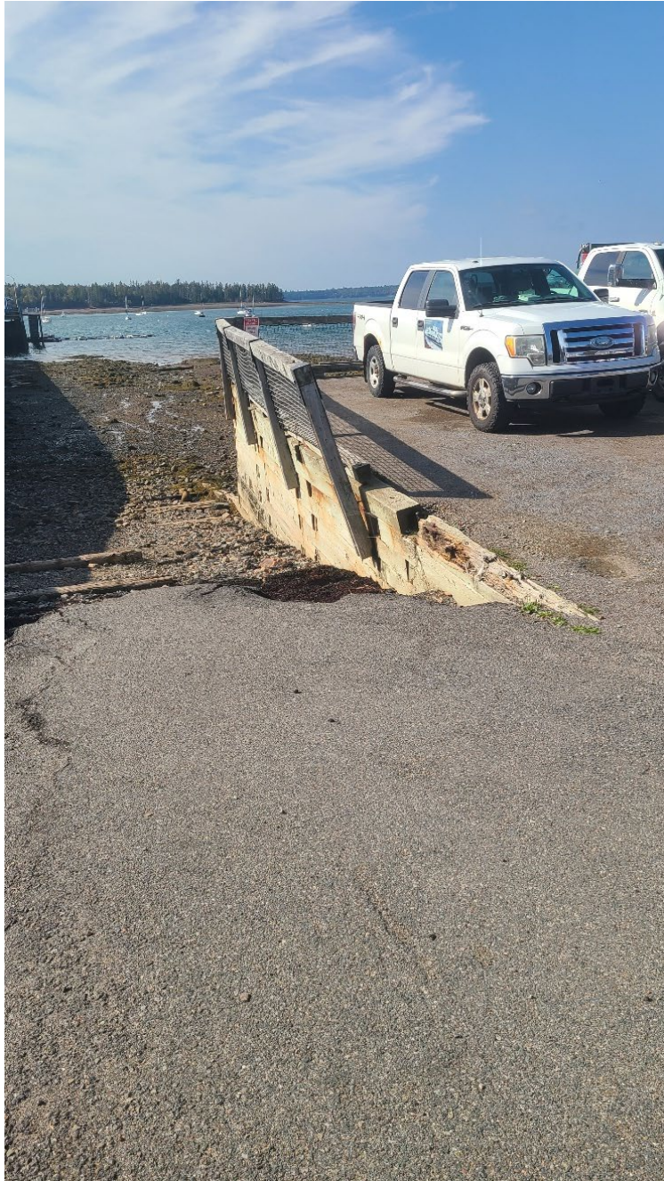
Figure 26: Crib Wall next to Shoreline Access.
