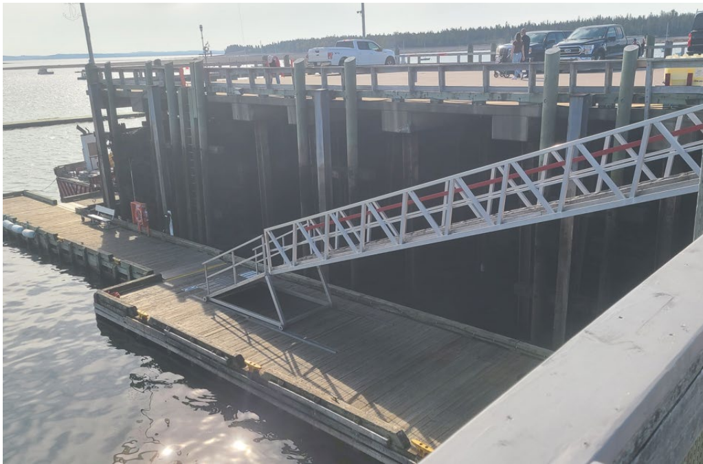
Figure 31: Eastern Gangway in Good Condition
